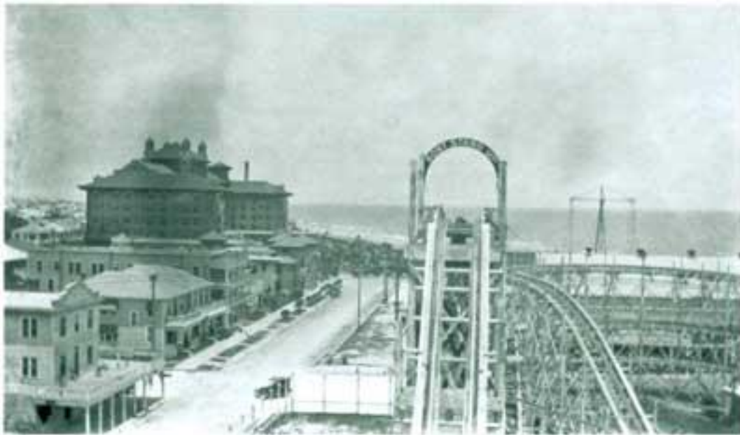
Above: an aerial view of the Mountain Speedway and the Buccaneer Hotel (under construction), circa 1929.
